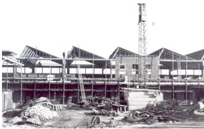
Construction of the conveyor belt hall
