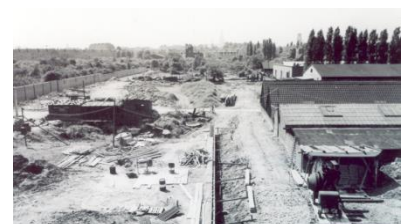
Extensions on southern firm area
