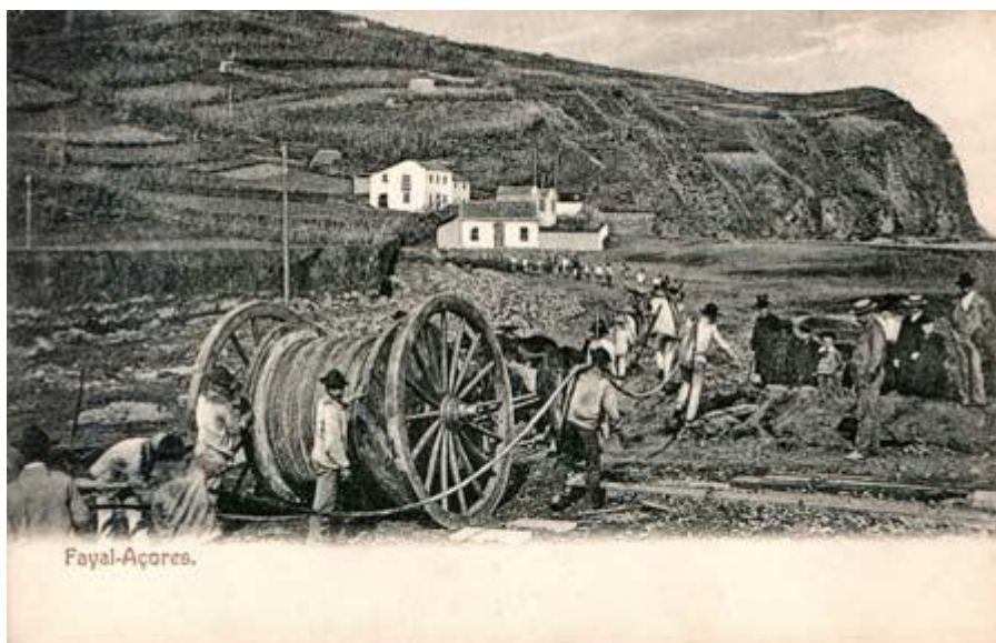
Laying cable from the Cable Hut to the Cable Station (date unknown).
