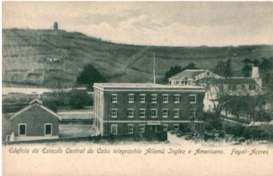
Joint Anglo, German and American Cable Station, Fayal, Azores
